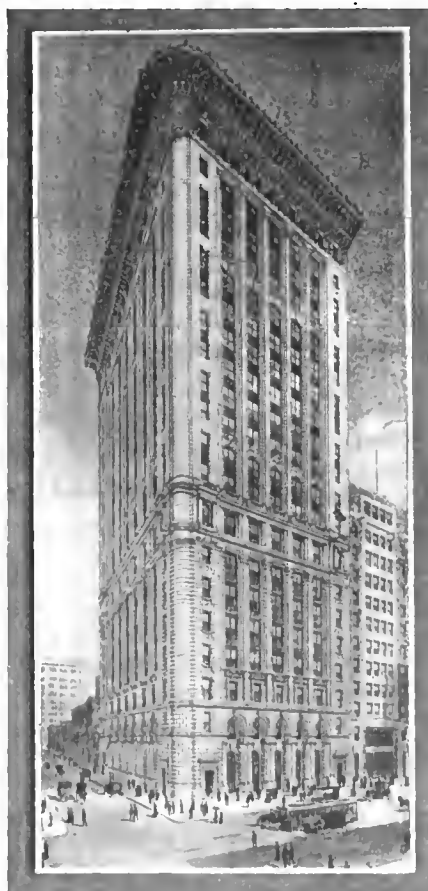
United States Rubber Company building now being erected in New York City
